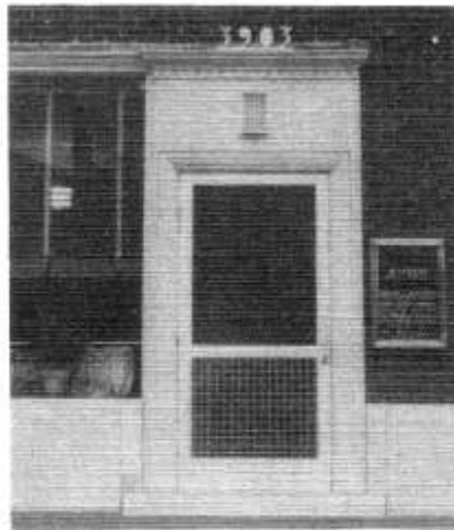
DOORWAY TO OFFICES ON SECOND FLOOR
