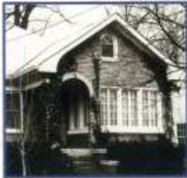
Mayor Nelson's House, 1950 - 1954 3957 Kennison Avenue
