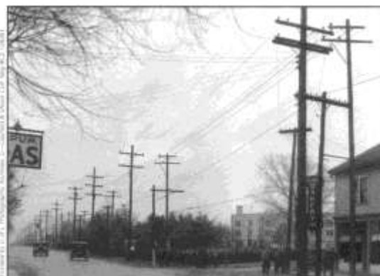
Looking east on Shelbyville Road in 1933 with Flehn's Bakery and Bethel Church in the background.
